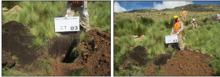
Calicata CT-03 - Km 2+800
